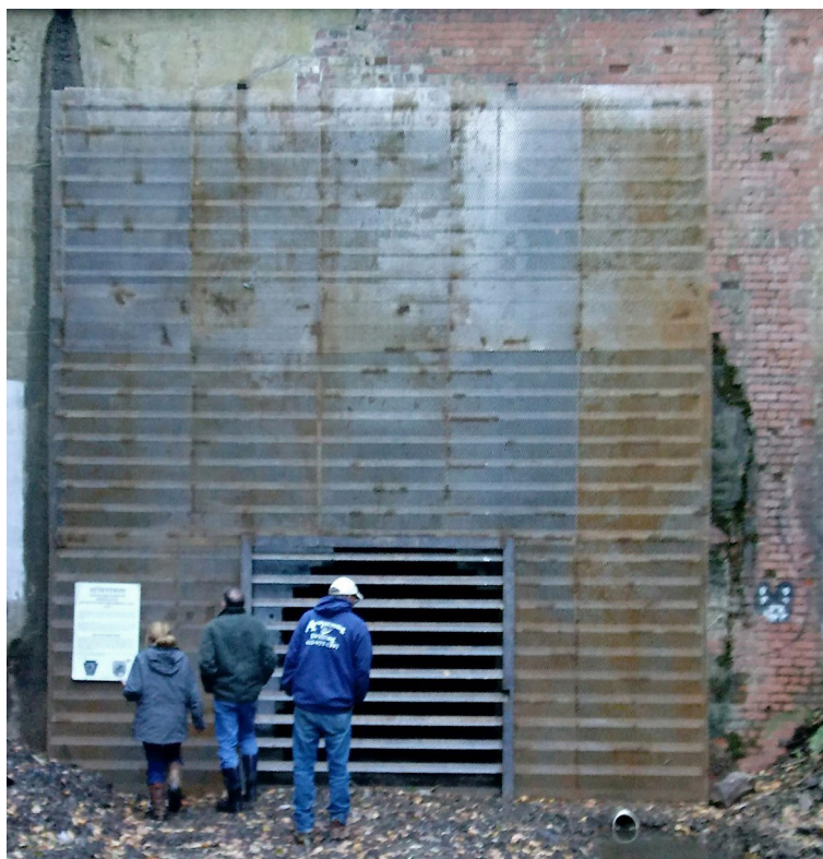
Completed gate to protect tunnel entrance.
